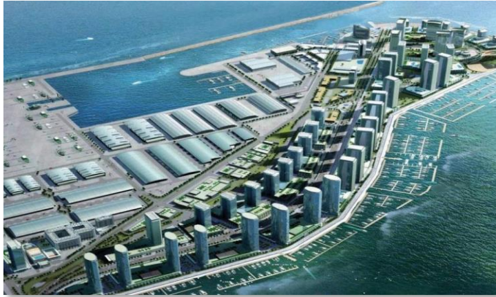
Purpose-build maritime centre, set to become a major hub for maritime services
