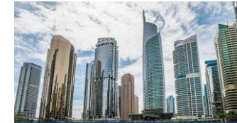
Jumeirah Lake Towers 150k RT
